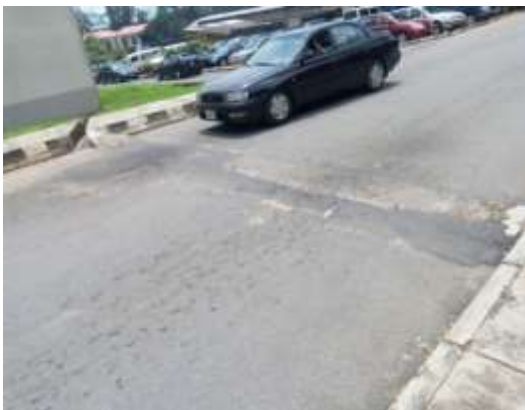
Figure 3: Speed hump made of concrete
