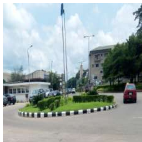
Figure 15: Typical Roundabout in the University of Ibadan
