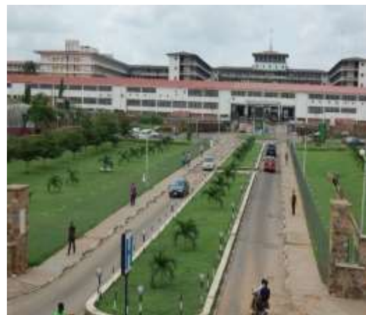
Figure 11: Well-maintained raised median in the Healthcare hub
