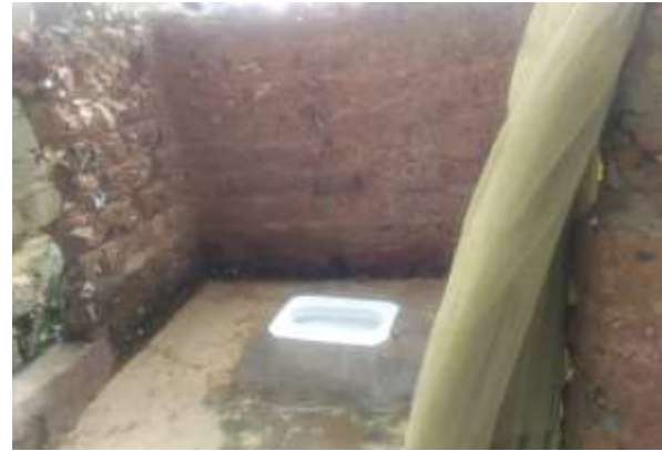
Plate 1: Mud block-built Toilet without roof at Sabon Tasha High Density Source: Author's Fieldwork, 2020
