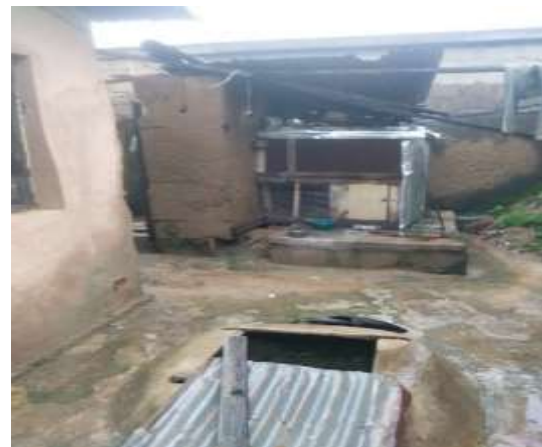
Plate 1.5: Safe distance of 2.3m between soakaway pit and well in Kawo high density Source: Author's Field survey, 2020.
