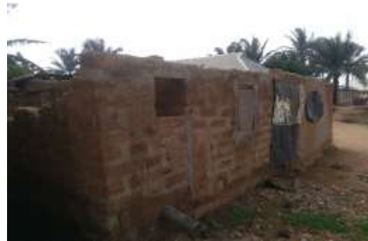
Plate 2: Mud block-built Toilet without roof at Unguwan Mu'azu/ Kabala West High Density Source: Author's Fieldwork, 2020.
